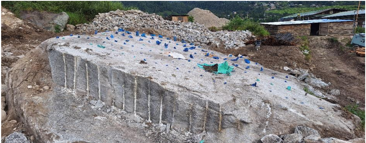
Photos 22-23: Field observations of ongoing construction works
