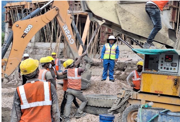
Photo 20: Discussions at control blasting site
