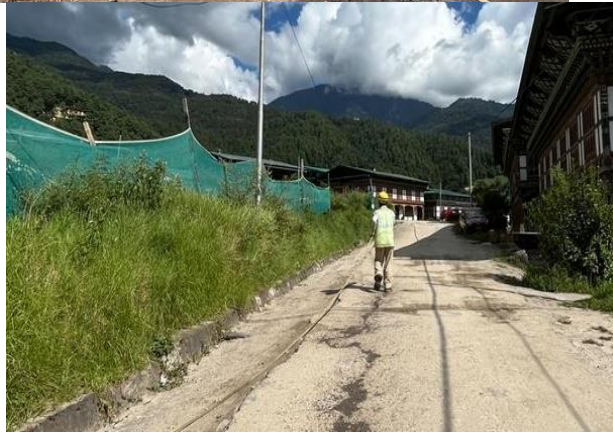
Photos 9-10: Spoil Disposal site
