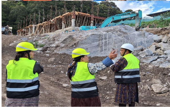
Photo 21: Control blasting of embedded rock at site. (Silent blasting using Aconex)
